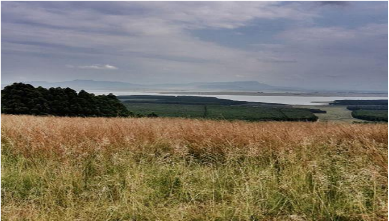
View of Heyshope Dam
